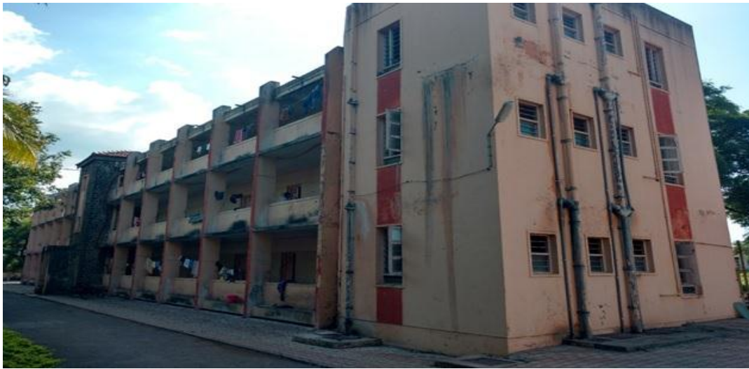
Fig. 1: Hostel building (D8) in WCE, Sangli.
