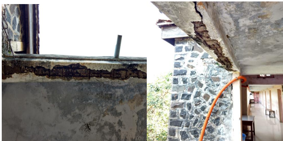
Fig. 4: Condition of Beams.
