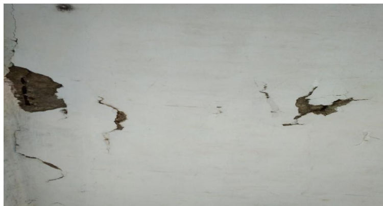
Fig. 6: Condition of slab.
