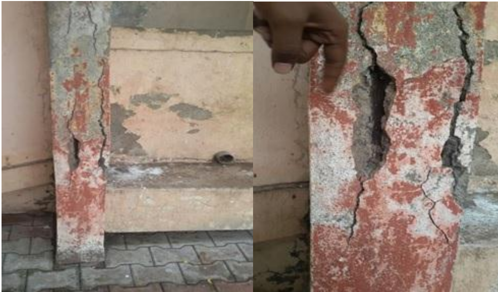
Fig. 3: Condition of Columns C2 and C13.
