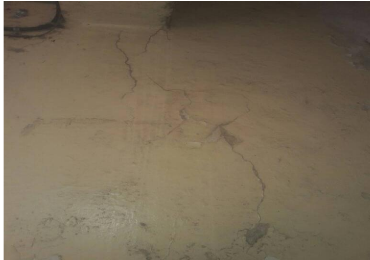
Fig. 5: Condition of wall.
