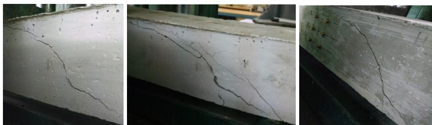
Figure 4: Cracks in reinforced concrete beams.
