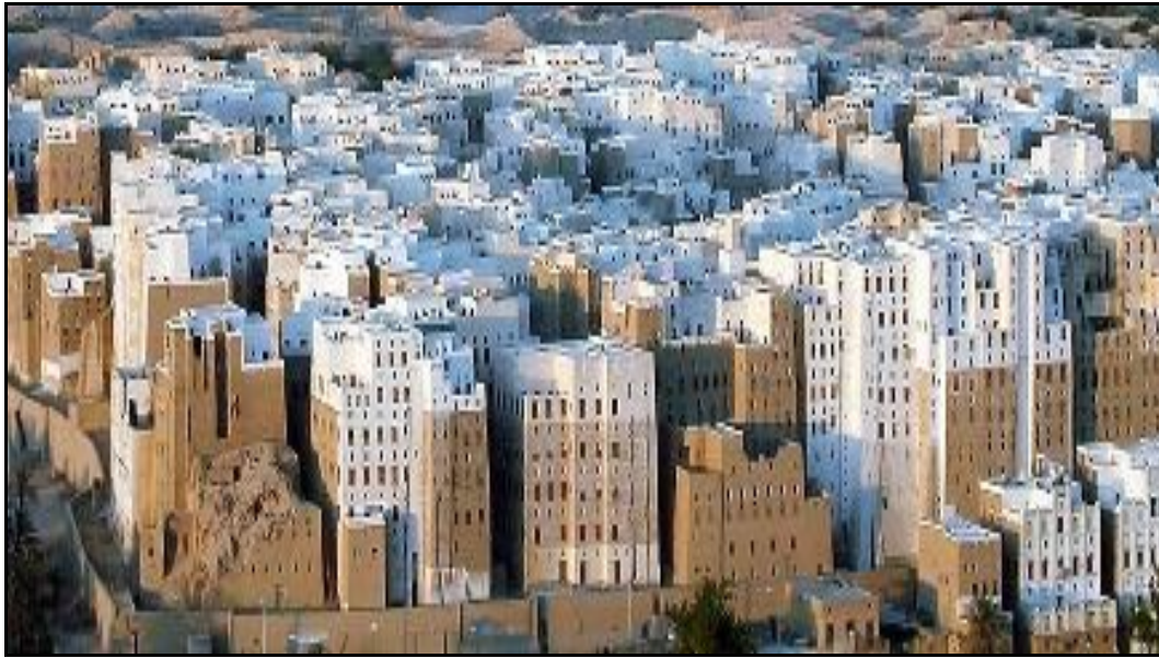
Figure 3: Illustrates View of Clay Buildings in the City of Shibam.
