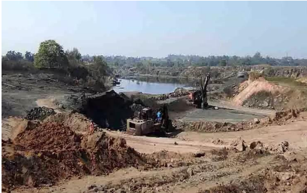
Figure 1: Operating Rajhara Colliery.
