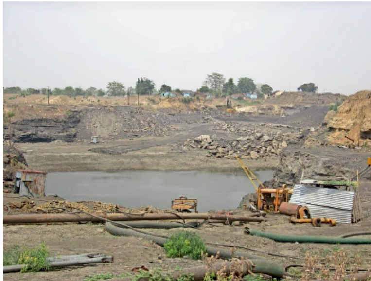
Figure 2: Rajhara coal quarry closed.
