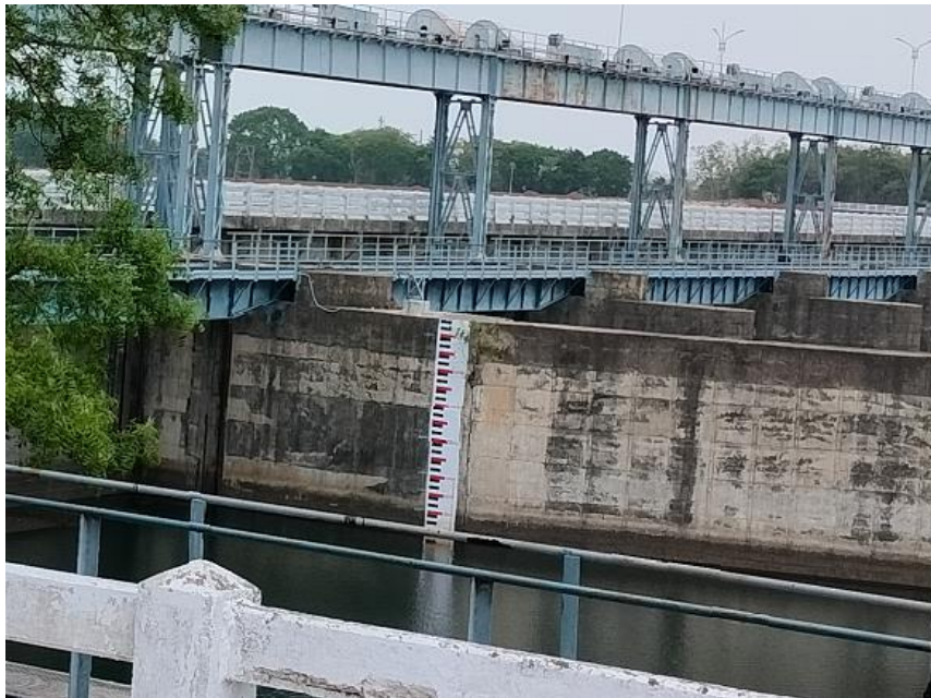
Figure 2: (Rudri Barrage, (District, Dhamtari) taken by me).
