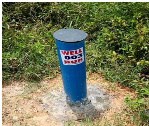
Fig. 1: Piezometer well for monitoring groundwater fluctuation.
