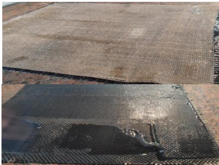
Fig. 12 Applying resin over fibers
