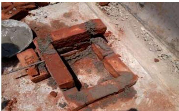
Figure 2: preparation of specimen to be plastered for thermo proof test.
