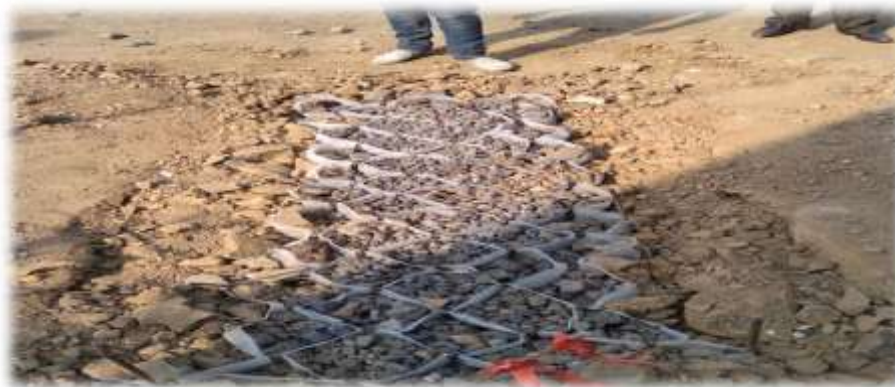
Fig no.3.11: Placing of Coarse aggregate.
