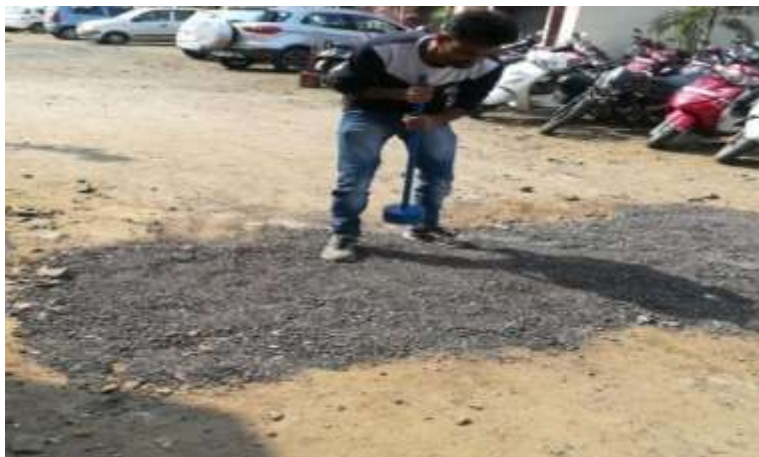
Fig no. 3.12: Compaction after placing.
