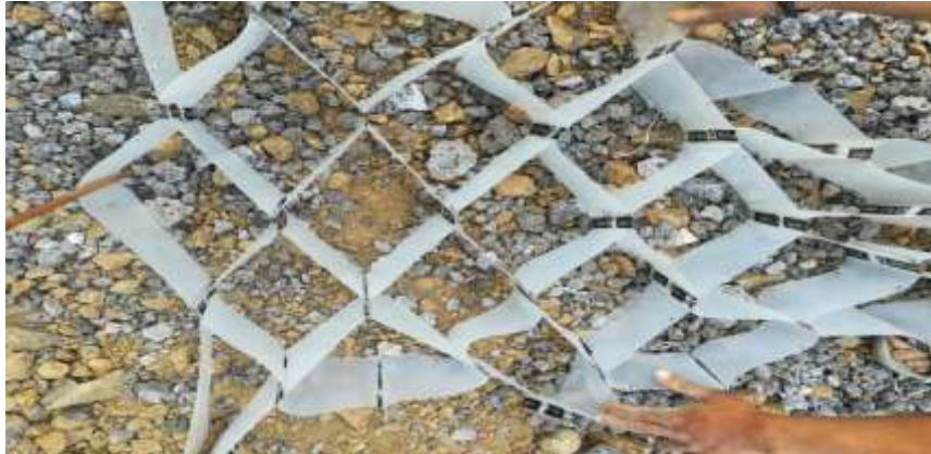
Fig no. 3.10: Placing of geocell.
