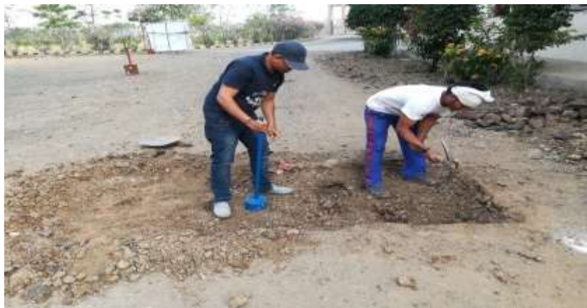
Fig no. 3.9: Compaction.
