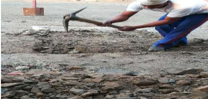
Fig no. 3.8: Excavation.
