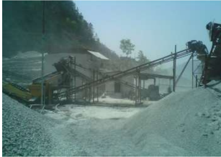
Fig 1: Crusher Plant, Kotre.
