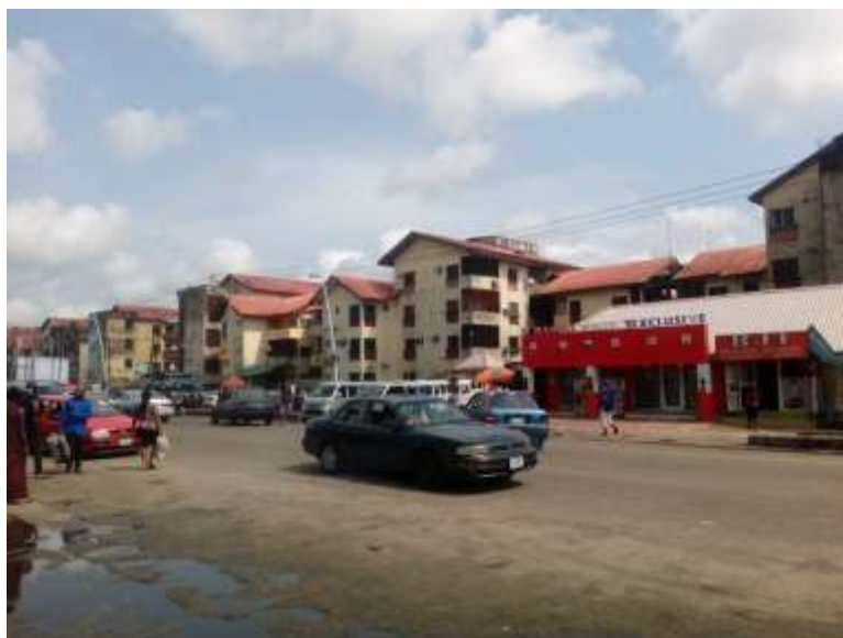
Fig. 1: Aggrey Road Housing Estate, Port Harcourt Municipality Source: Researcher's Field Survey, 2018.
