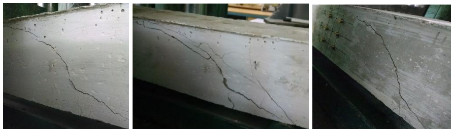
Figure 4: Cracks in reinforced concrete beams.
