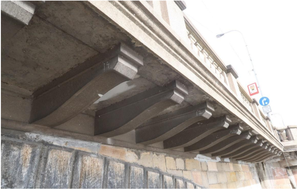
Figure 6: View of the bridge widening.
