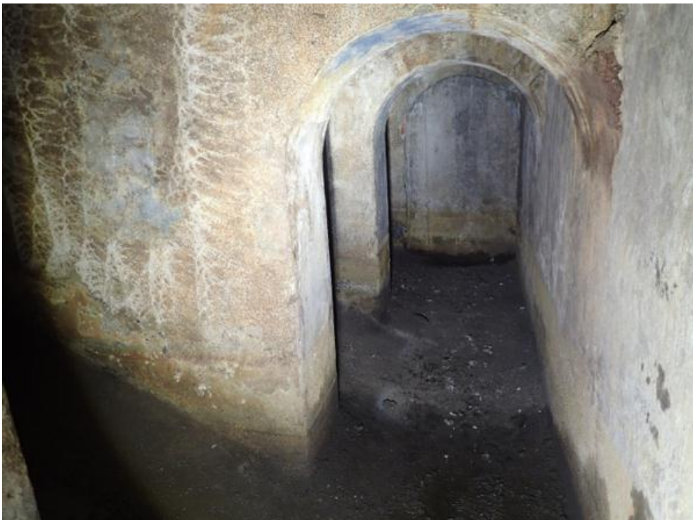
Figure 7: View into the relief chamber.
