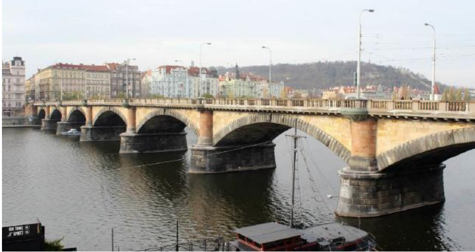
Figure 1: View of the bridge.
