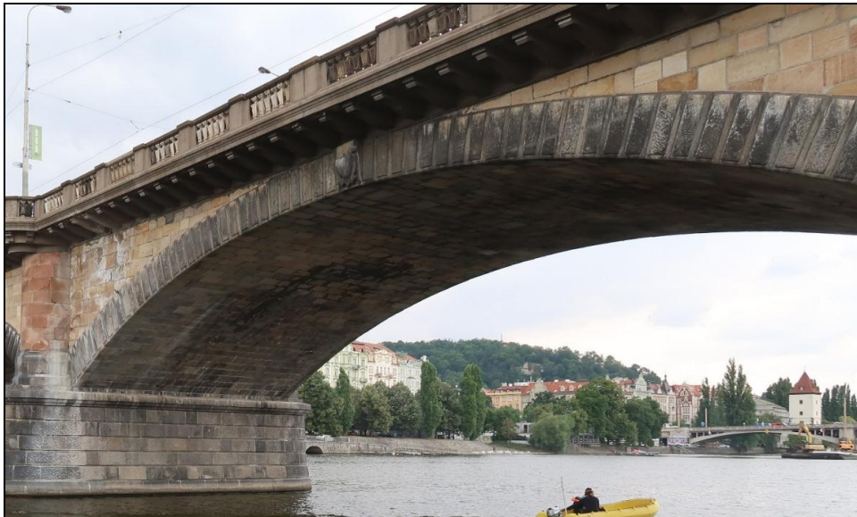
Figure 2: Stone arch of the bridge in detail.
