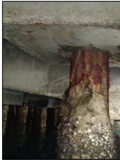
Figure 1: Photo of Corroded Reinforced Concrete Pile.
