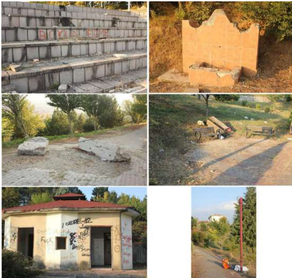
Fig. 5: Some examples vandalism Duzce, Turkey (Original, 2015).
