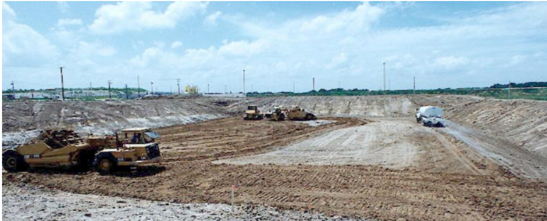
Figure 1: Showing cement stabilised subgrade at test site.
