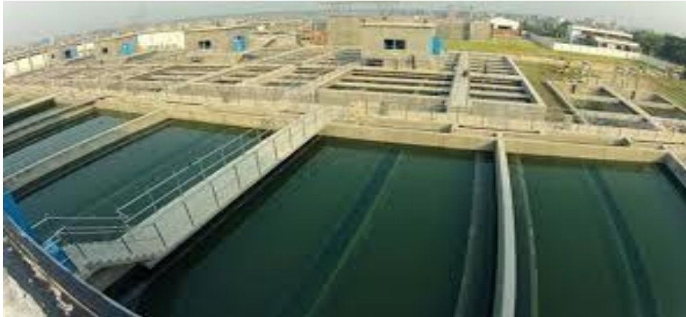
Figure 12: Installation of Surface water treatment plant for Mongla Port Authority.
