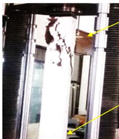
Figure 4 Failure mechanism of the unstrengthened Reference RC column NC1.
