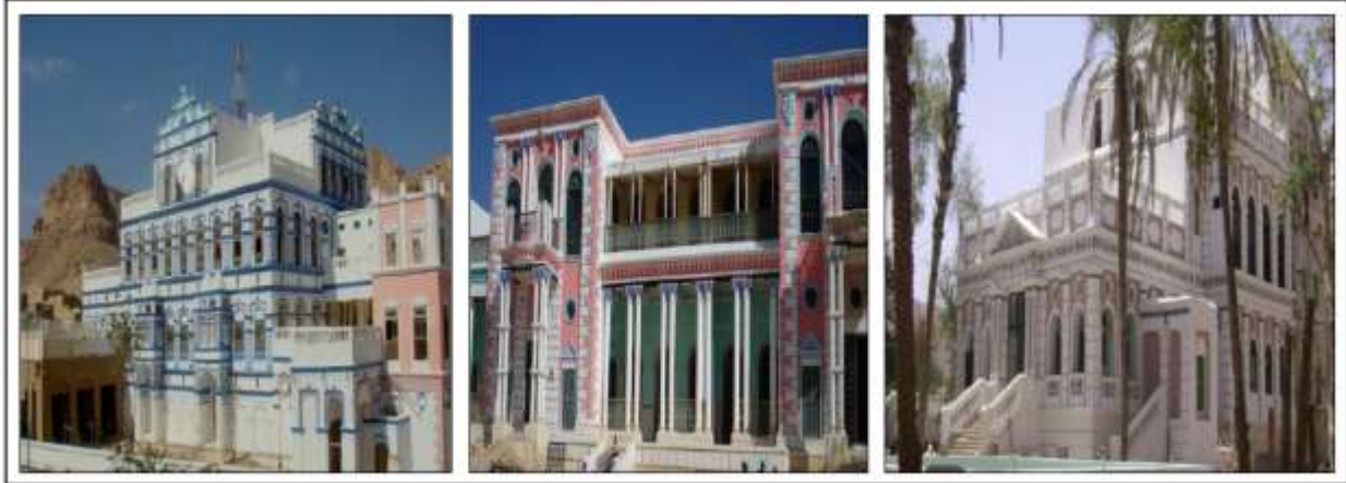
Figure 4: Architectural Style of Clay Buildings in Hadhramout Region.
