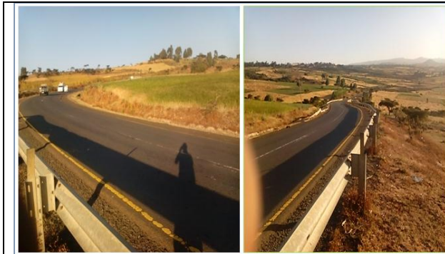
Figure 3.10: Minini Existing Road Condition.
