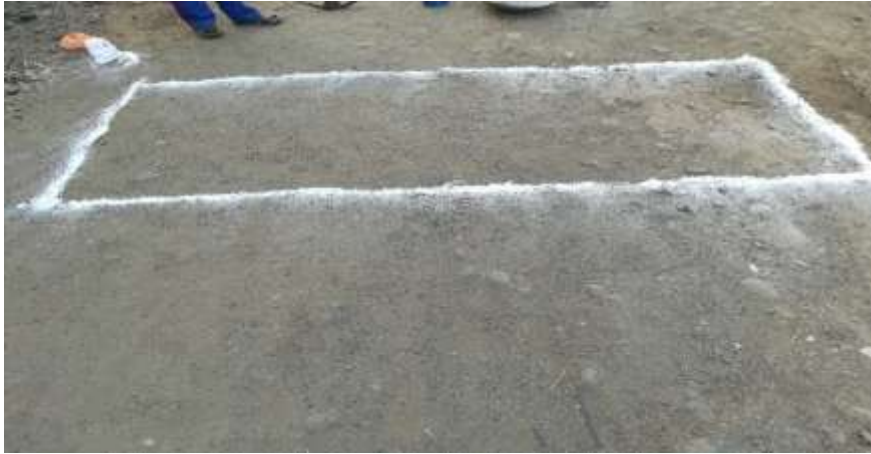
Fig no. 3.7: Test Patch.
