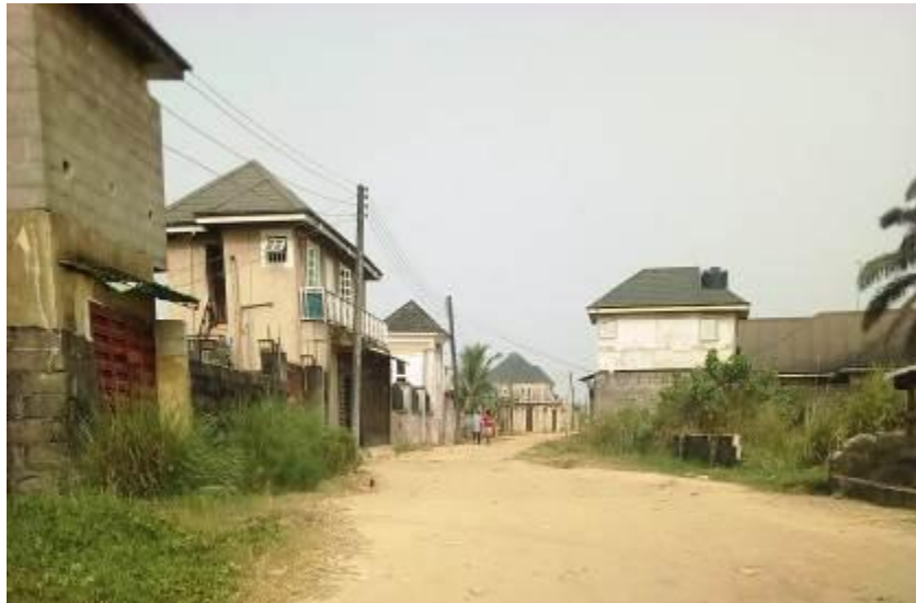
Plate 1: Ozuoba – Road without drainage.
