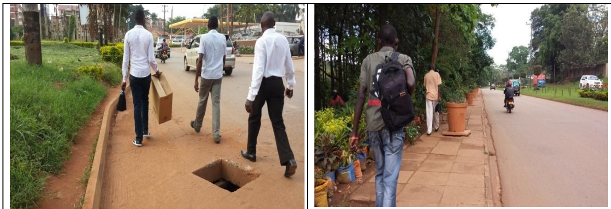
Figure 3: Risky open manhole along Luthuli Avenue and flower pots along Yusuf Lule Road.
