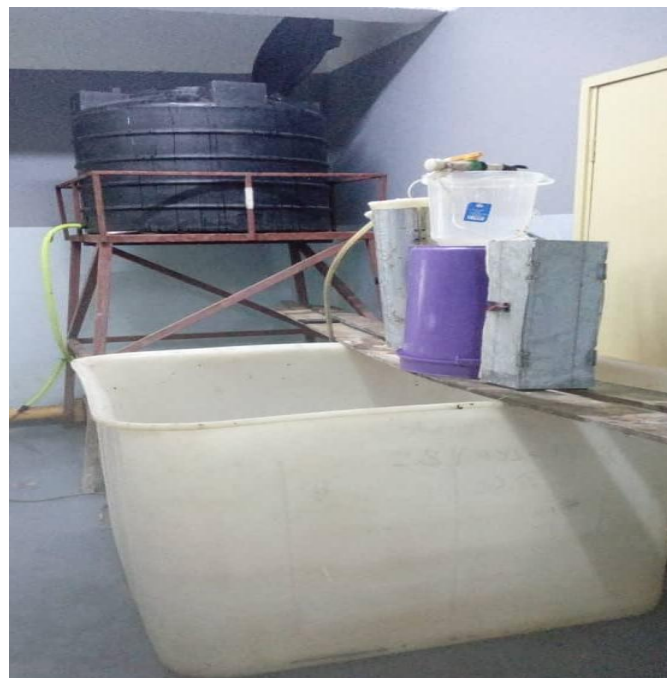
Figure 9: Enhanced curing technique of vertical concrete members using water reservoir.
