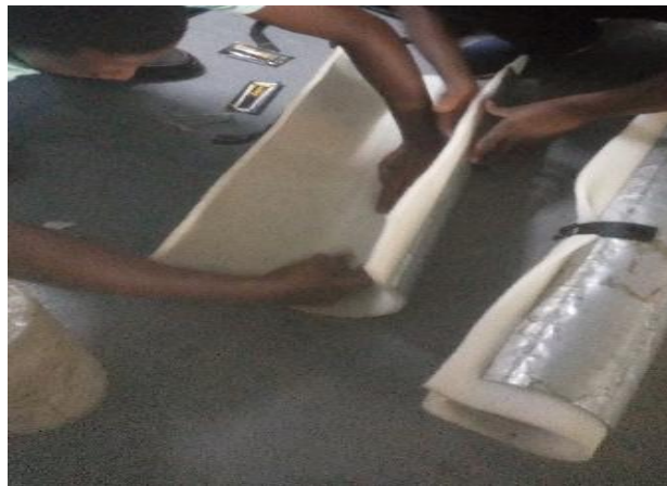
Figure 8: Fabrication of the membrane.
