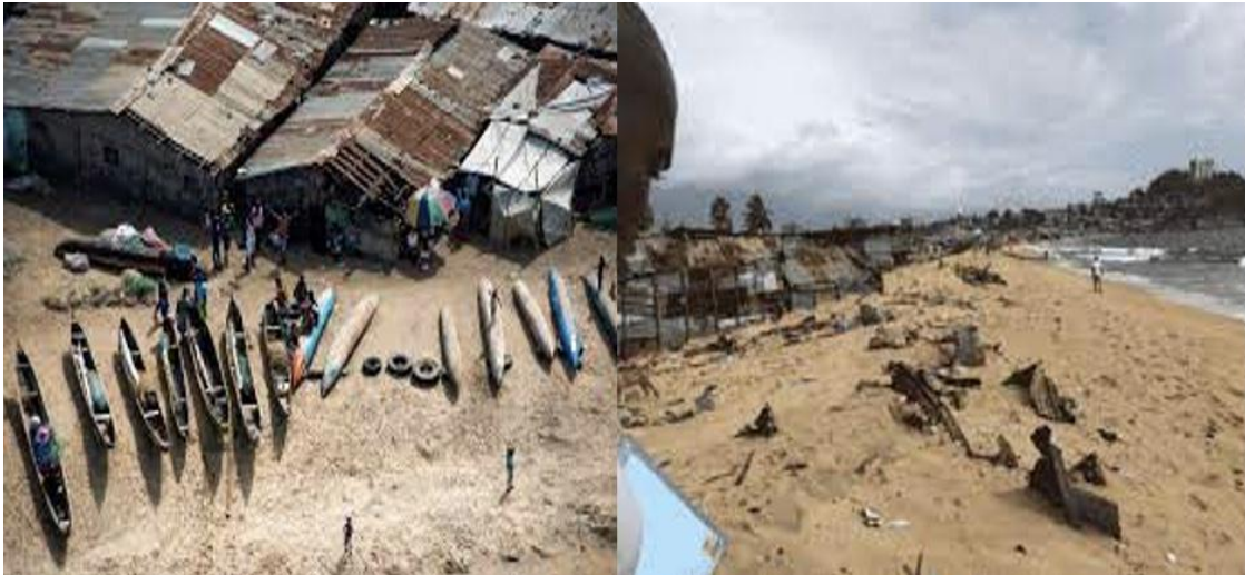
Figure 5: Merged images of Near Sea West Point and Infrastructure in New Kru Town.
