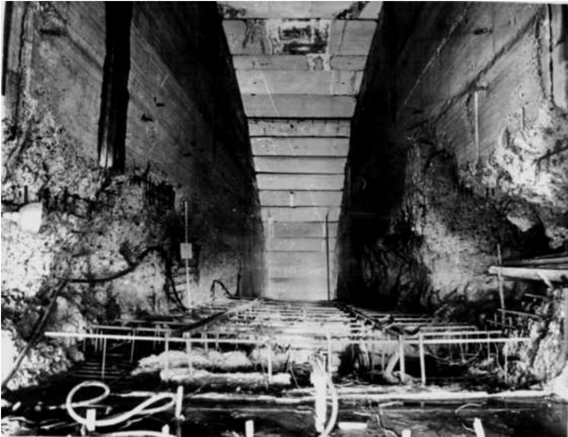
Figure 4: Sayano-Shushenskaya HPP (Russia). Construction spillway of the second tier. Cavitation-induced damages to the floor and sidewalls behind the gate chamber (1980).
