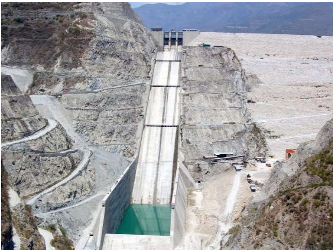
Figure 19: Surface flow of the Teri HPP (India), equipped with aerator trampolines.
