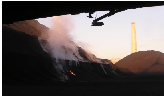
Figure 2: Fire in a coal pile at Rutenburg Coal Fired Power Station, Ashkelon, Israel (March, 2003)
